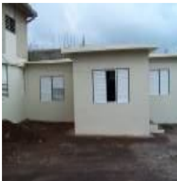
Completed storage area
